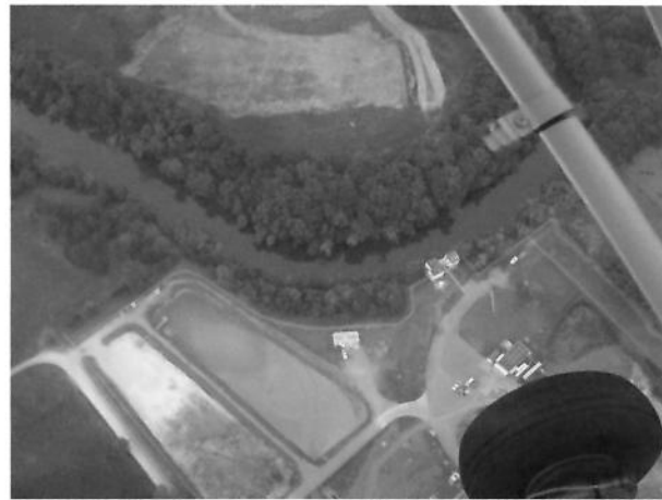
water treatment plant at bottom edge of landfill on top
